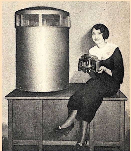
The idea for the huge Diesel air-silencer at the left was inspired by the auto silencer easily held by the woman on the right. It filters and cleans the air entering the motor.
