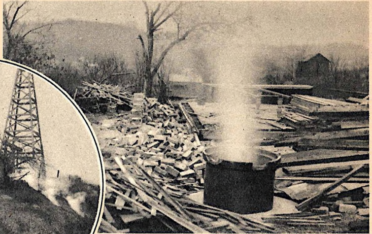
Overnight cistern of this home became belching smokestack for raging coal fire far below, compelling owner to tear down home, piece by piece, and move it hurriedly to more solid location.
