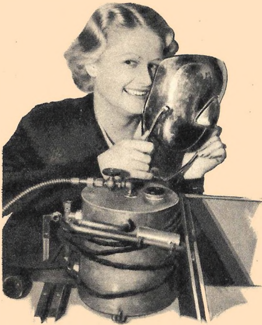
The metal mask is moulded to fit the face. Medical ingredients are heated to the vapor point in the electric unit. Vapor passes to the mask to be emitted through pin-holes in lining.
