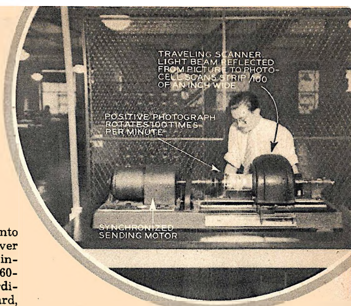
To get photos in newspapers simultaneously with press association stories, Associated Press has developed Wirephoto service to send pictures by wire. Photocell scans photo, sends impulses over wire to similar receiving machine which has light-valve that acts on sensitive negative. After being developed, print is made and half-tone cut prepared for newspaper.
