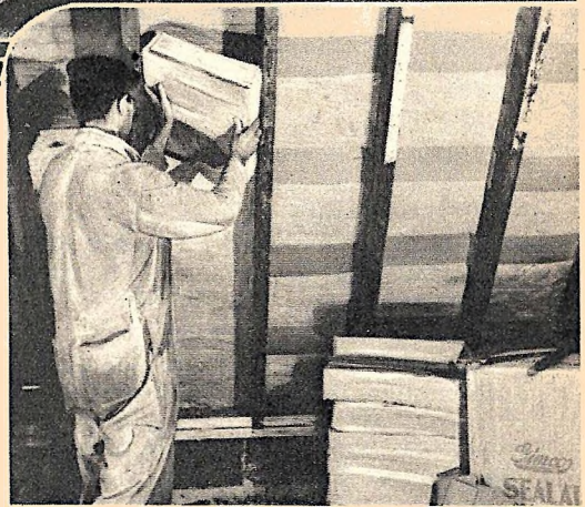
Blankets for the house roof and walls, such as the above, are made from limestone, slag, glass and other materials to reduce heat losses and keep out summer temperatures.
