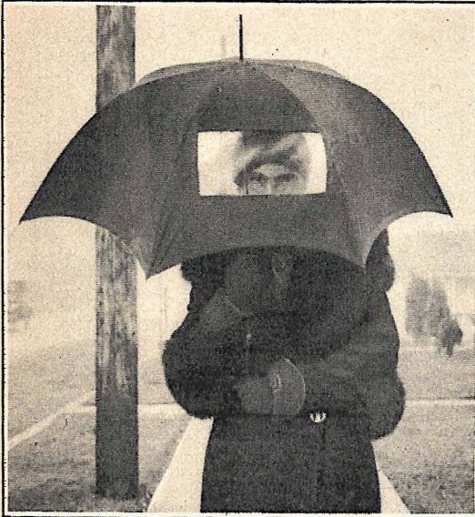
The new umbrella window consists of a piece of isinglass set into the front to afford the user clear vision ahead.
