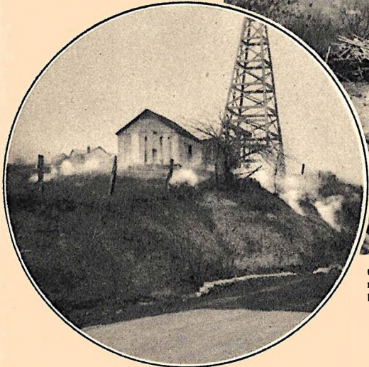
Though underground fire is burning all around, this oil well near New Straitsville, Ohio, is still producing. Road suddenly sank five feet here (at darker part) and had to be filled in.
