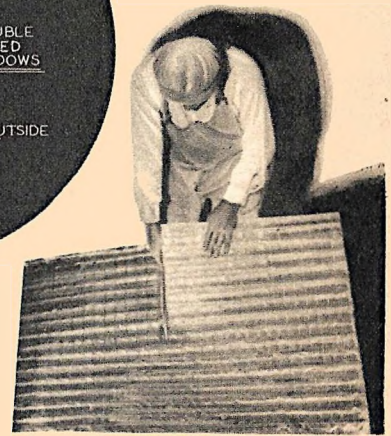
Above—New double-paned window reduces loss of heat. Right—Aluminum lath material has reflecting heat side and dull side for plaster.
